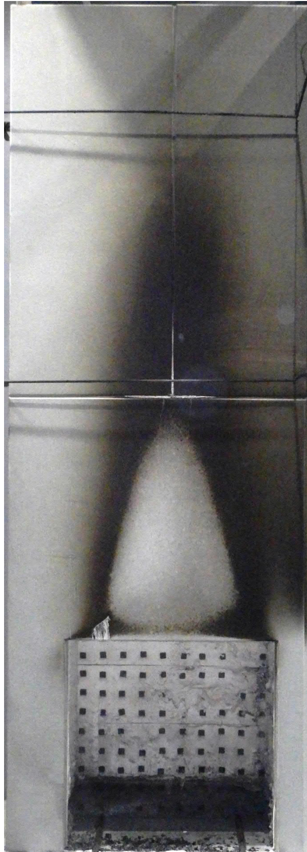
Figure 33 The external wall system on completion of the test – main wall
