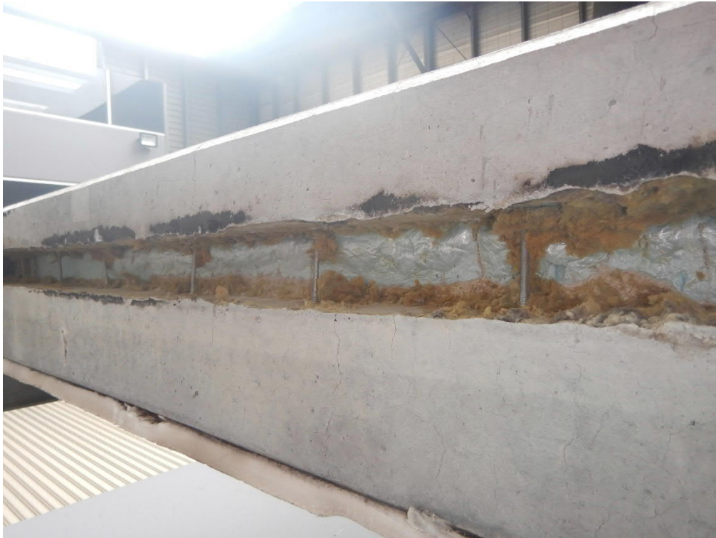
Figure 35 Condition of insulation behind the stone wool layer above the opening, with the stone wool removed
