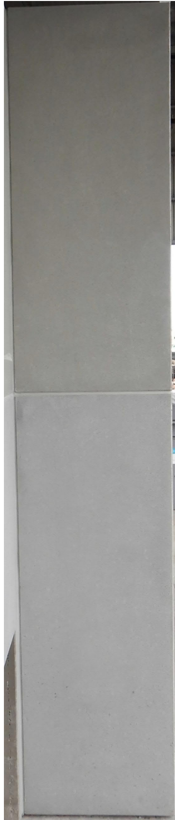
Figure 25 The external cladding system before the start of the test – wing wall
