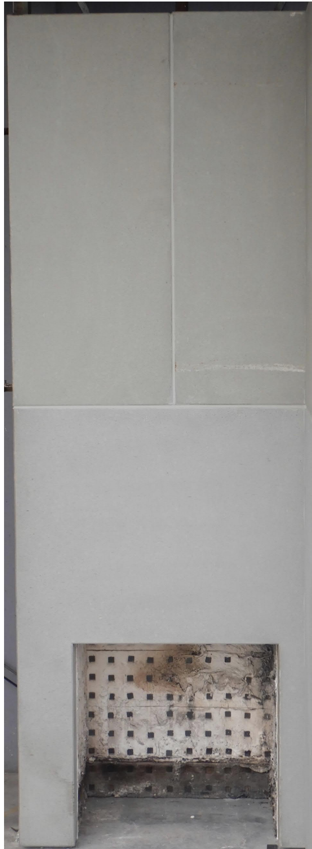
Figure 24 The external cladding system before the start of the test – main wall
