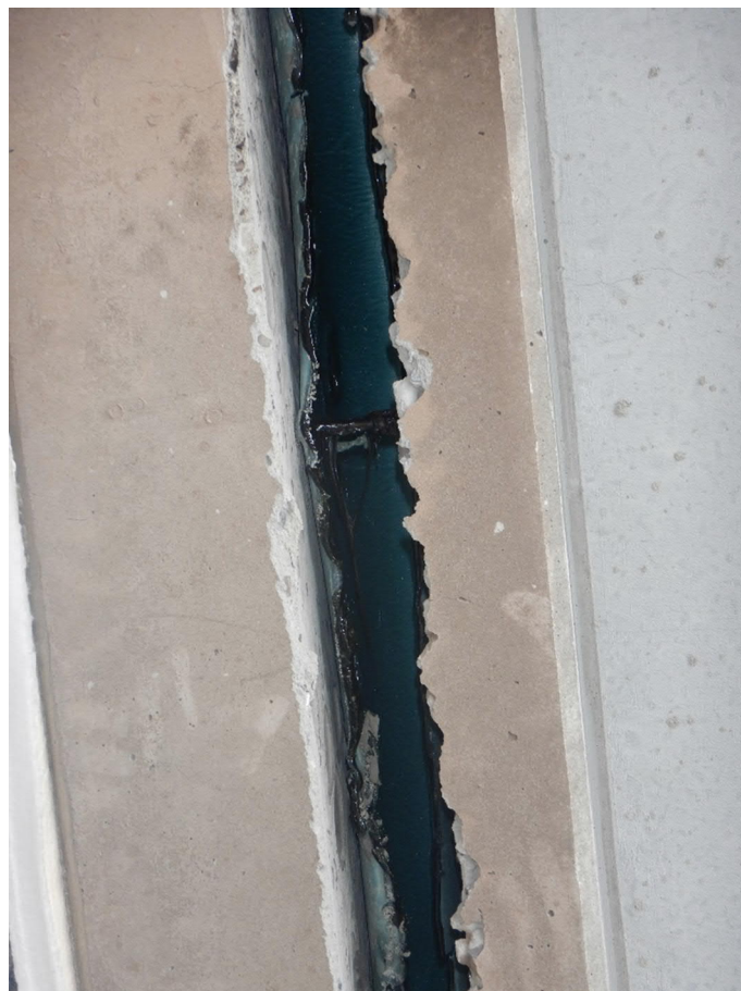
Figure 35 Condition of insulation behind the stone wool layer above the opening, with the stone wool removed
