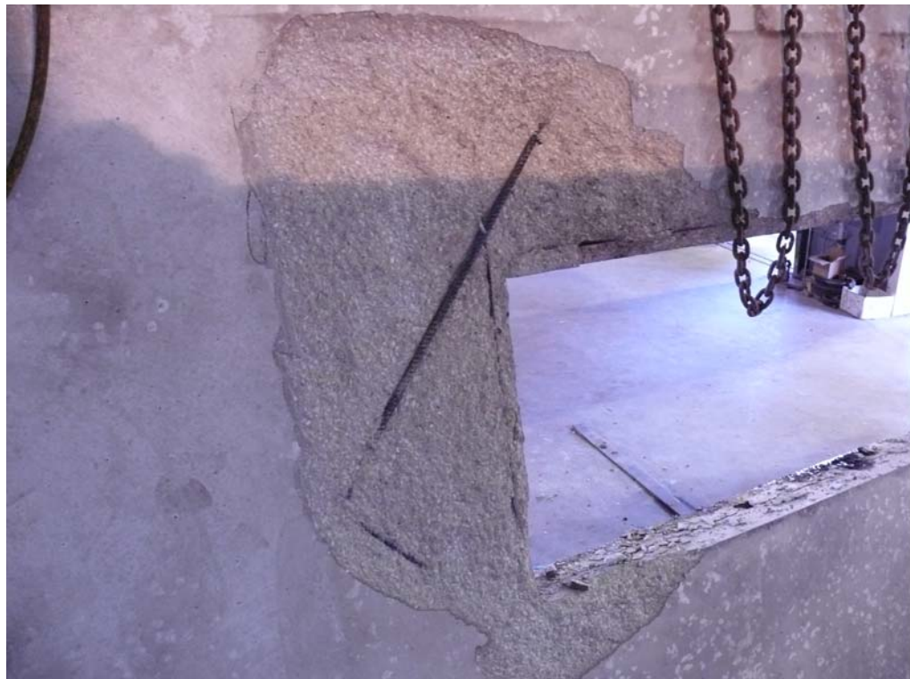
Figure B-4. Interior Face – Post Test Inspection.
