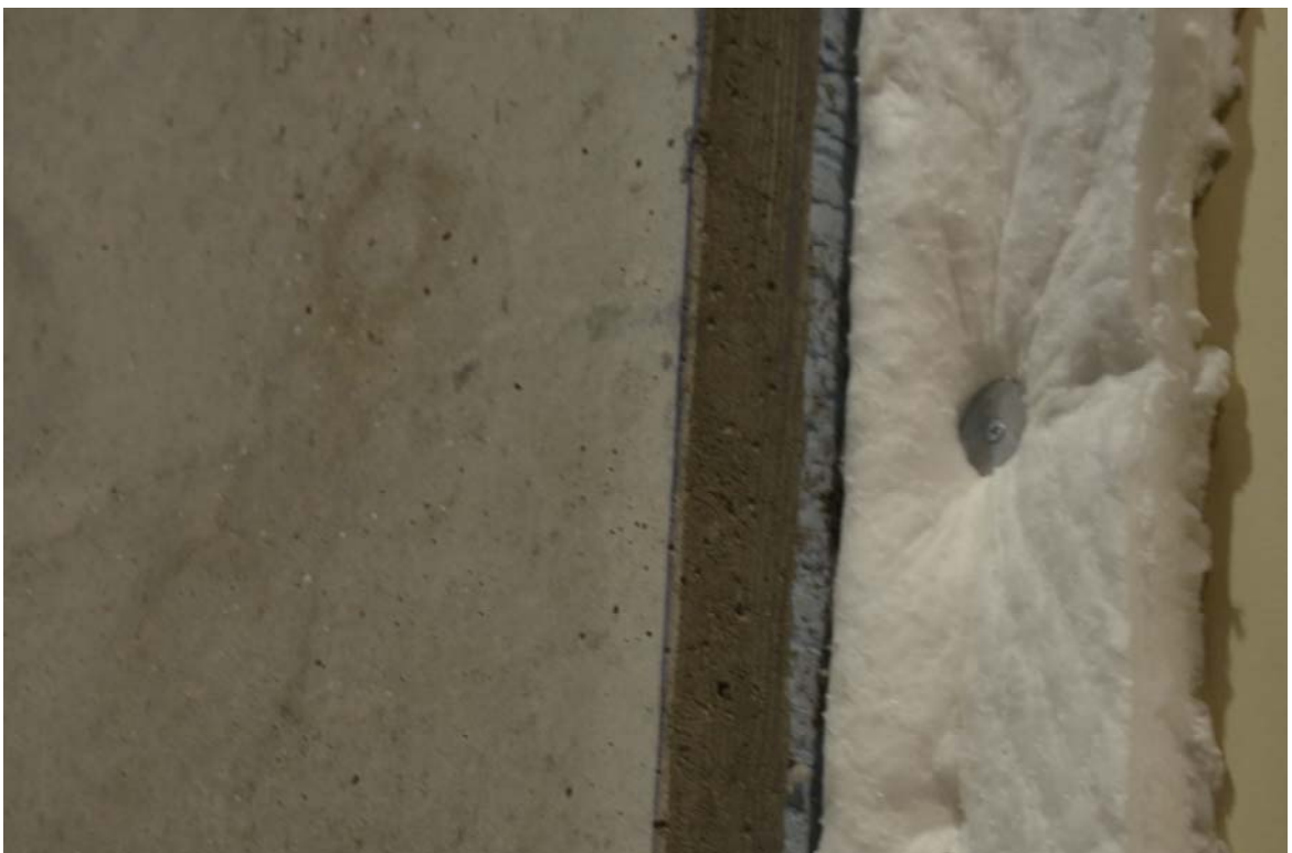
Figure B-2. Close-Up of Unexposed Side of Wall prior to Testing.
