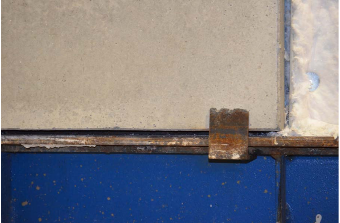
Figure B-3. Close-Up of Unexposed Side of Wall prior to Testing Showing Steel Clip.
